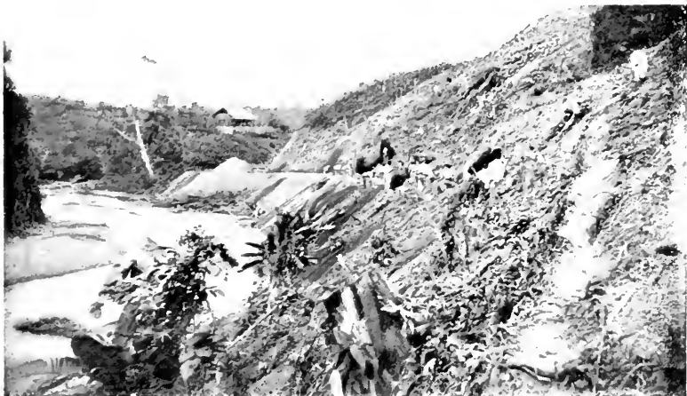
SIDE-HILL CUT NEAR BELLA VISTA.
